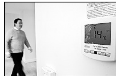
KEEP COOL: The temperature in the eco-home is carefully controlled
